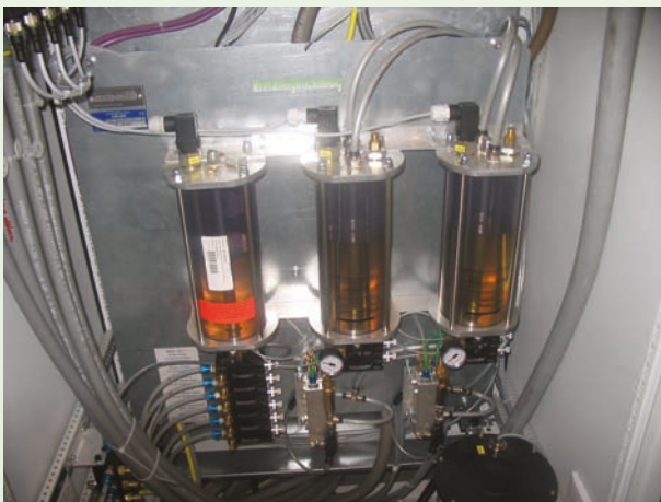
6 pumps for outside lubrication 4 pumps for inside lubrication
