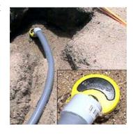
per day. About 65% of indoor use occurs in the bathroom and 1/3 of that flushes down the toilet. The Green House reclamation system collects and filters grey water from sinks, showers, baths, laundry and the yard for reuse in toilets and irrigation. The system includes a 120 gallon underground water cistern. EchoPod measures the level, and opens the fill valve to replenish the system with tap water, if necessary.
